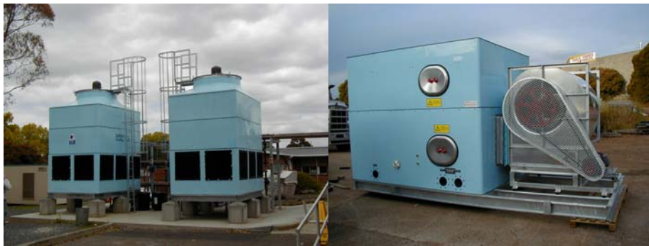
Figure 3. Induced Draft and Forced Draft Cooling Tower.
