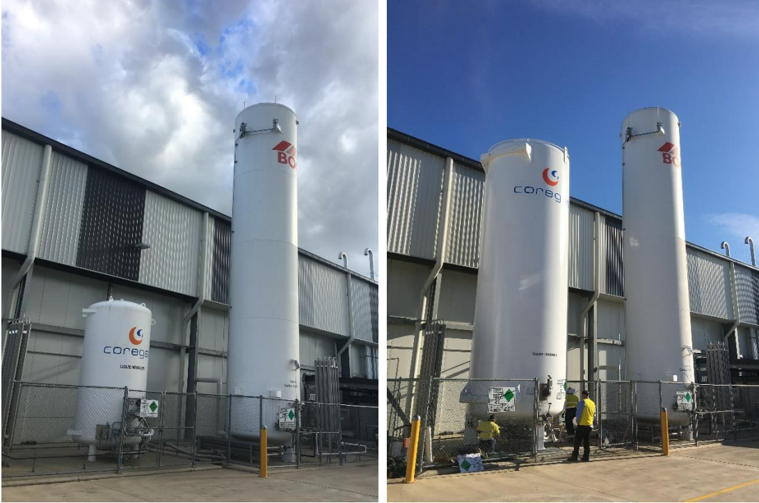
Photo 17: Nitrogen storage tank before and after
