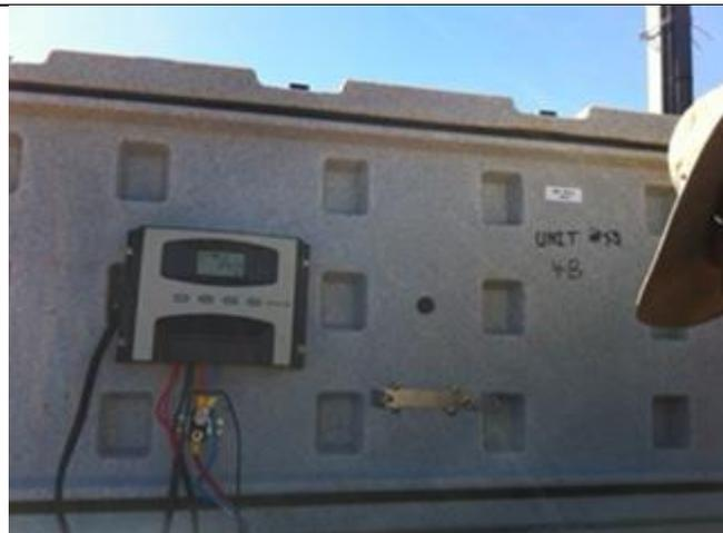
**Figure 11.5b. Voltage regulator that moderates incoming solar power to charge battery. When these fail the battery is rapidly destroyed**
