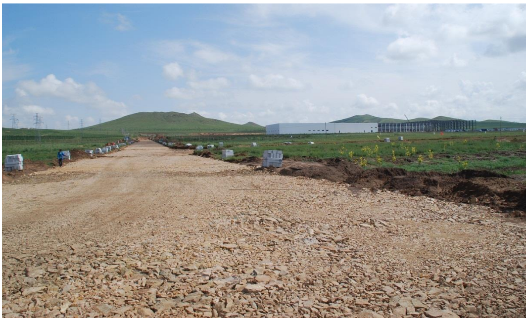
Fig. 13 The entrance to the new processing centre in Xilinhot.
