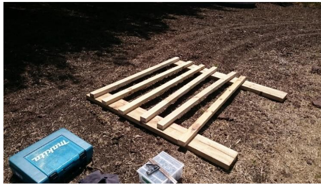
Figure 8 - Laying out the timber ready to construct a timber panel to match the portable cattle panels at site 2
