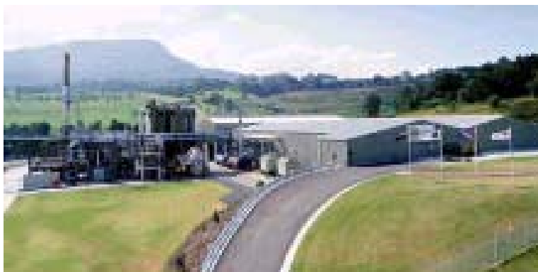
Figure 18 SWERF plant, Wollongong
