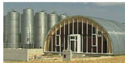
Figure 121 Biodiesel Plant in Austria
