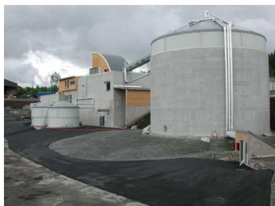
Figure 12 Exterior of the finished plant
