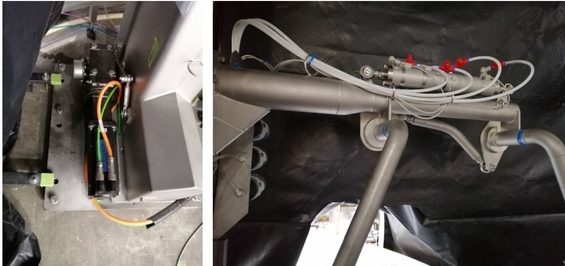
Figure 20: Lifter arms during the build phase – Fabrication and assembly completed successfully without notable issue.
