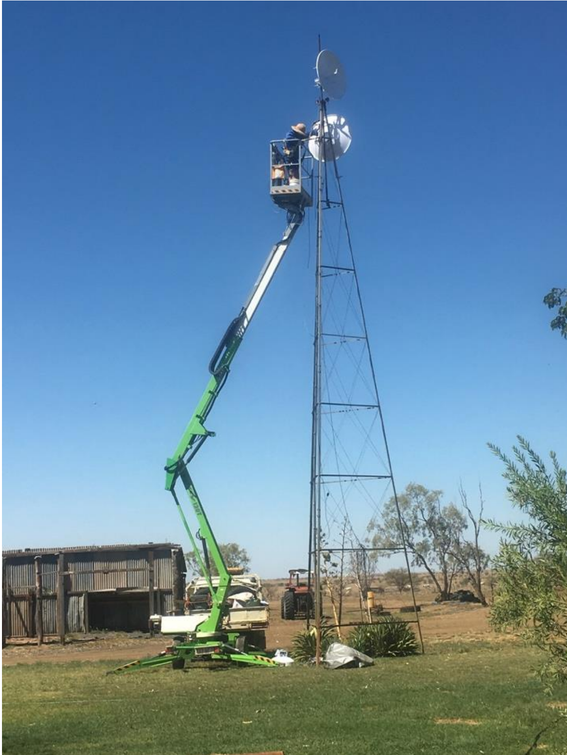
Photo 5: Final alignment of dish commissioned on the tower located at Essex.
