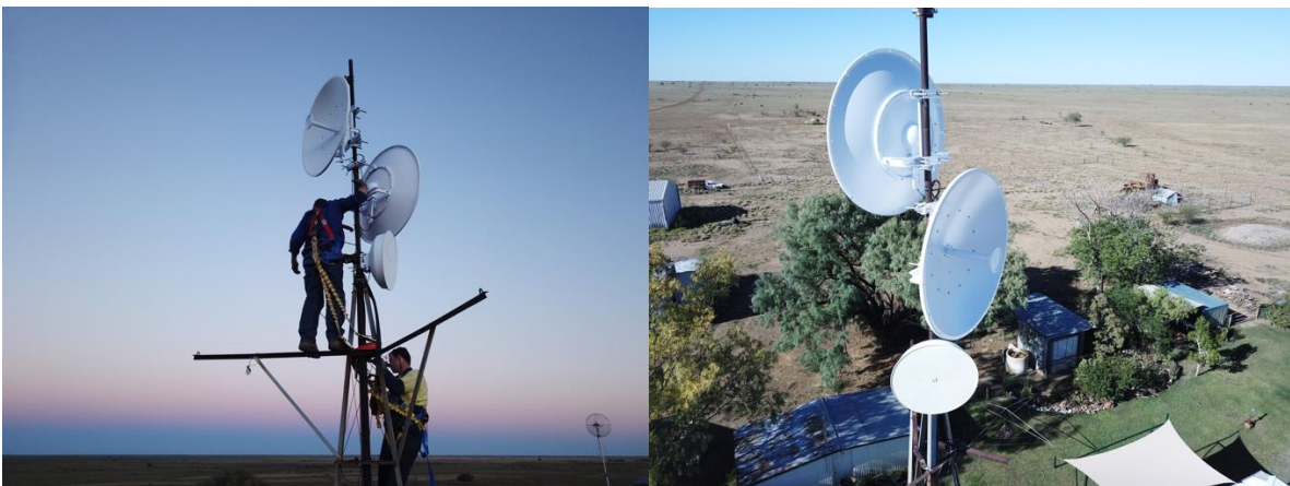
Photo 7: Final alignment of the Bernborough
