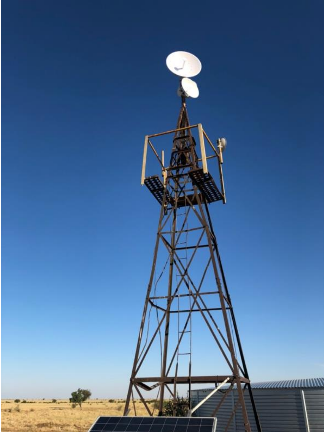
Photo 8: Tower construction at station.
