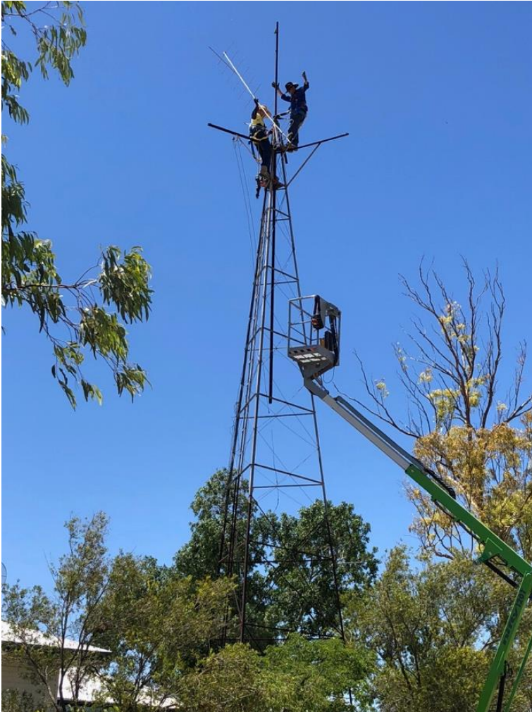
Photo 6: Tower under construction at Bernborough.
