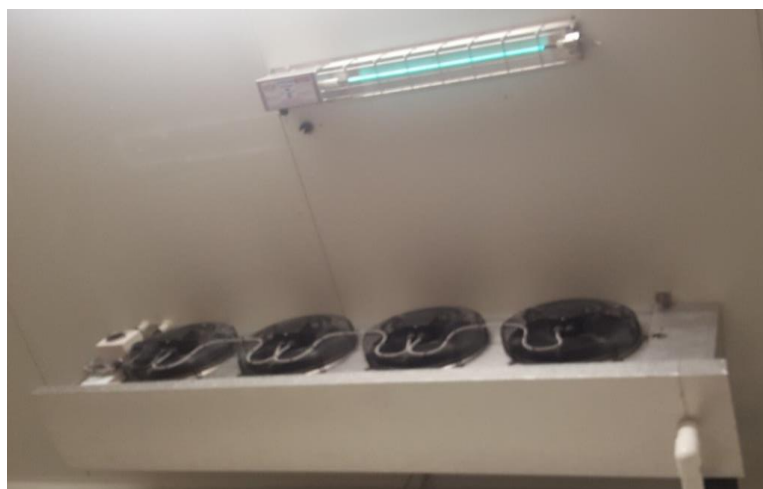
Figure 20. Chamber evaporator & operating UV unit
