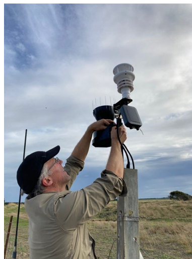
Figure 2 - Installation of weather station
