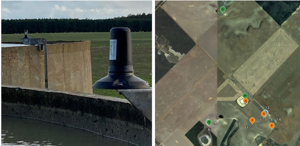
Figure 37 - Waterwatch sensors on two Coolindown Farms water tanks
