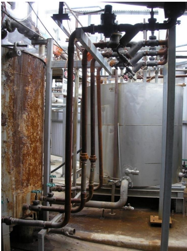
82°C steam sparge system with original tanks
