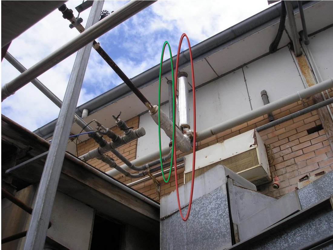
Steam and condensate lines entering and leaving the boning room
