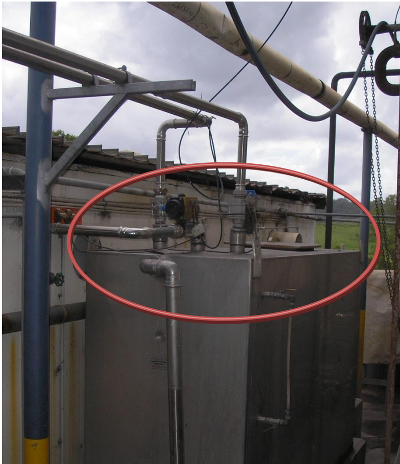
Boiler softener feed water tank with control valves indicated
