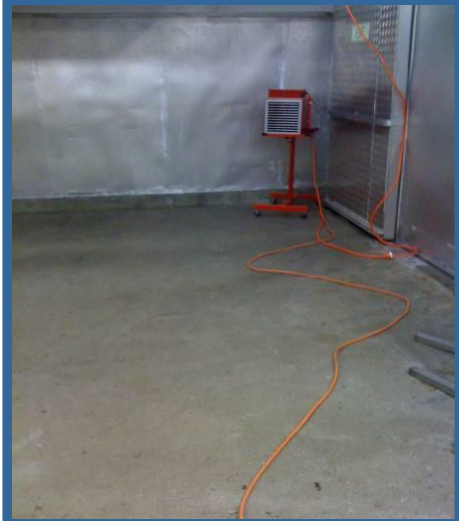
FIGURE 2. Hotbox-Axial Blower Heater HB90415—415V 9.0kW in small chiller B - dry floor post heating.
