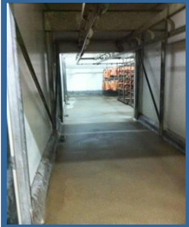
FIGURE 4: (a) Large chiller A showing bollards, floor wall coving with exit door open to holding chiller with product in the distance and (b) same chiller with exit door shut and showing overhead framework.
