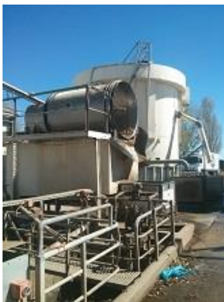
Photo 1: Existing Contra-shear in foreground with DAF at rear.
