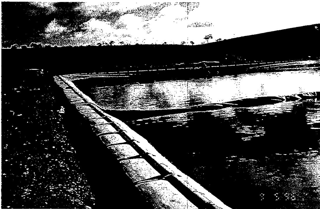
Photo 7. View of Lagoon 1 showing baffle (centre) and biogas collection header (perimeter of lagoon) prior to cover installation
