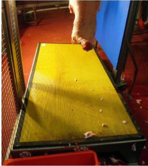
Fig. 9 Safety mat at carcass entry point
