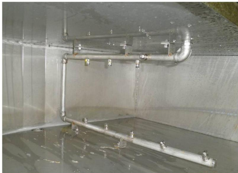
Fig.11 Wash tank nozzle configuration
