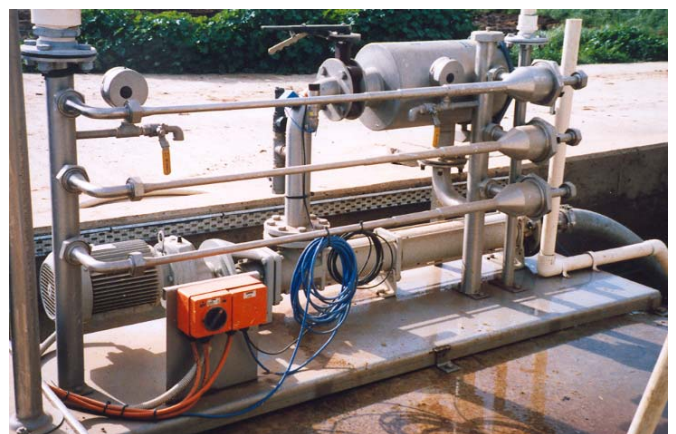
Figure 10 Meat Processing Plant No.3 – Hydrocyclone Installation
