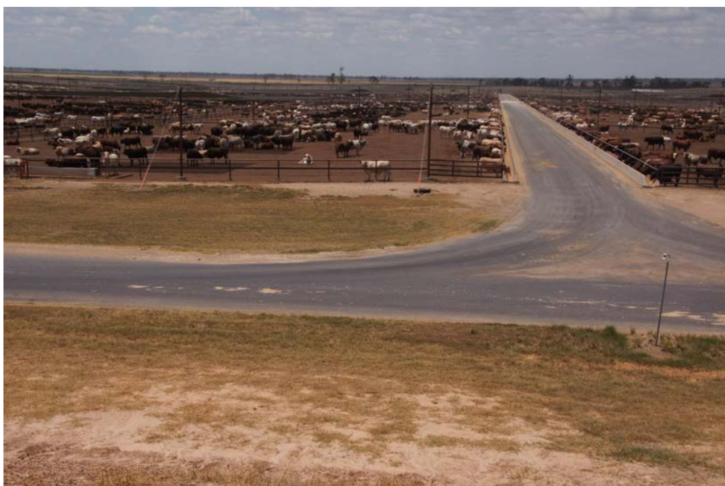
Photograph 18 – Bitumen sealed roads eliminate traffic-generated dust
