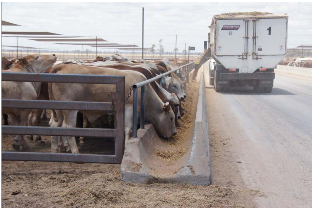
Photograph 17 – Sealed feed road eliminates dust to cattle when feeding
