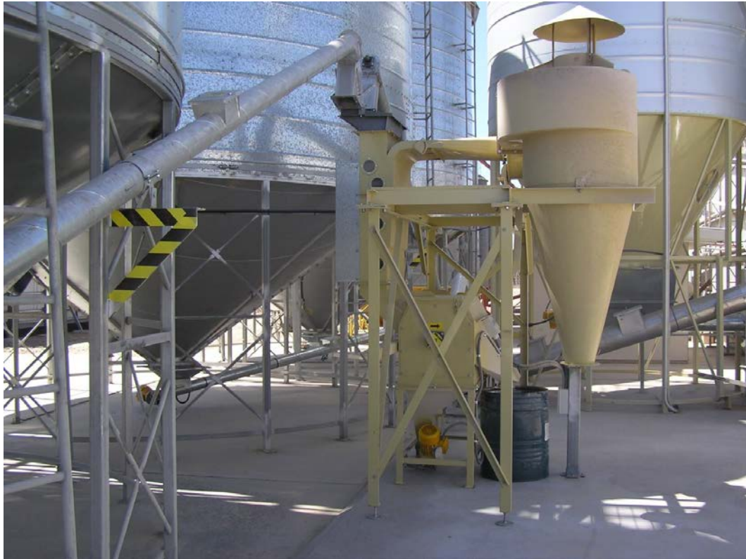
Photograph 24 – Grain scalper and cyclone to remove dust
