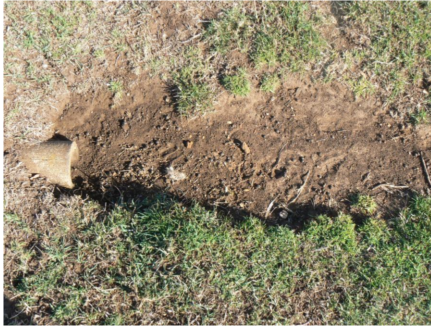
Fig. 5. A down pipe outlet showing a bare area that never supports plant life.
