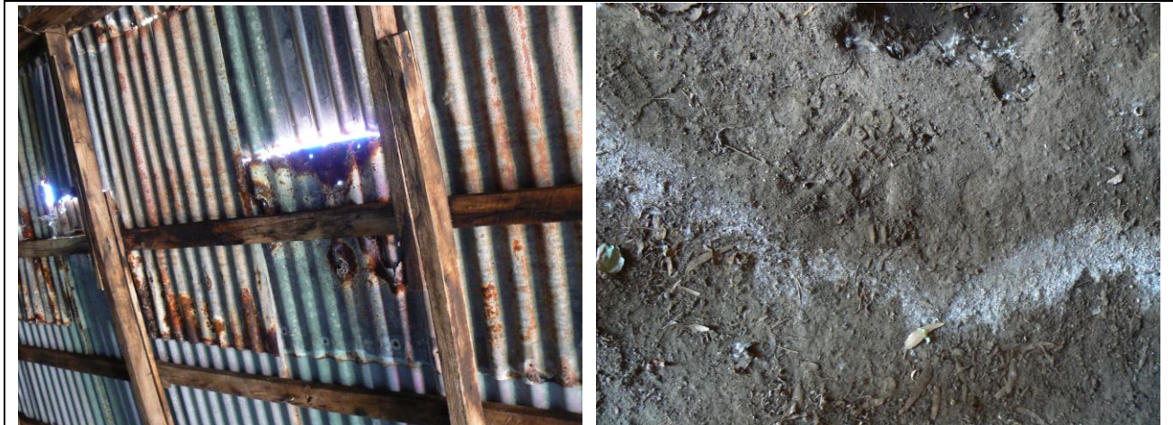
Fig. 6. Photo A. shows the corroded section of the corrugated iron roof overlap, on a typical old farm shed allowing dew and rain to leak onto the dirt floor below. Photo B. An aerial view showing the dirt floor below the leaky roof. In the upper area of the photo is the drip zone, the area adjacent and below it is the wet zone, the central white area is a calcium deposit, bordered below by the dry zone.
