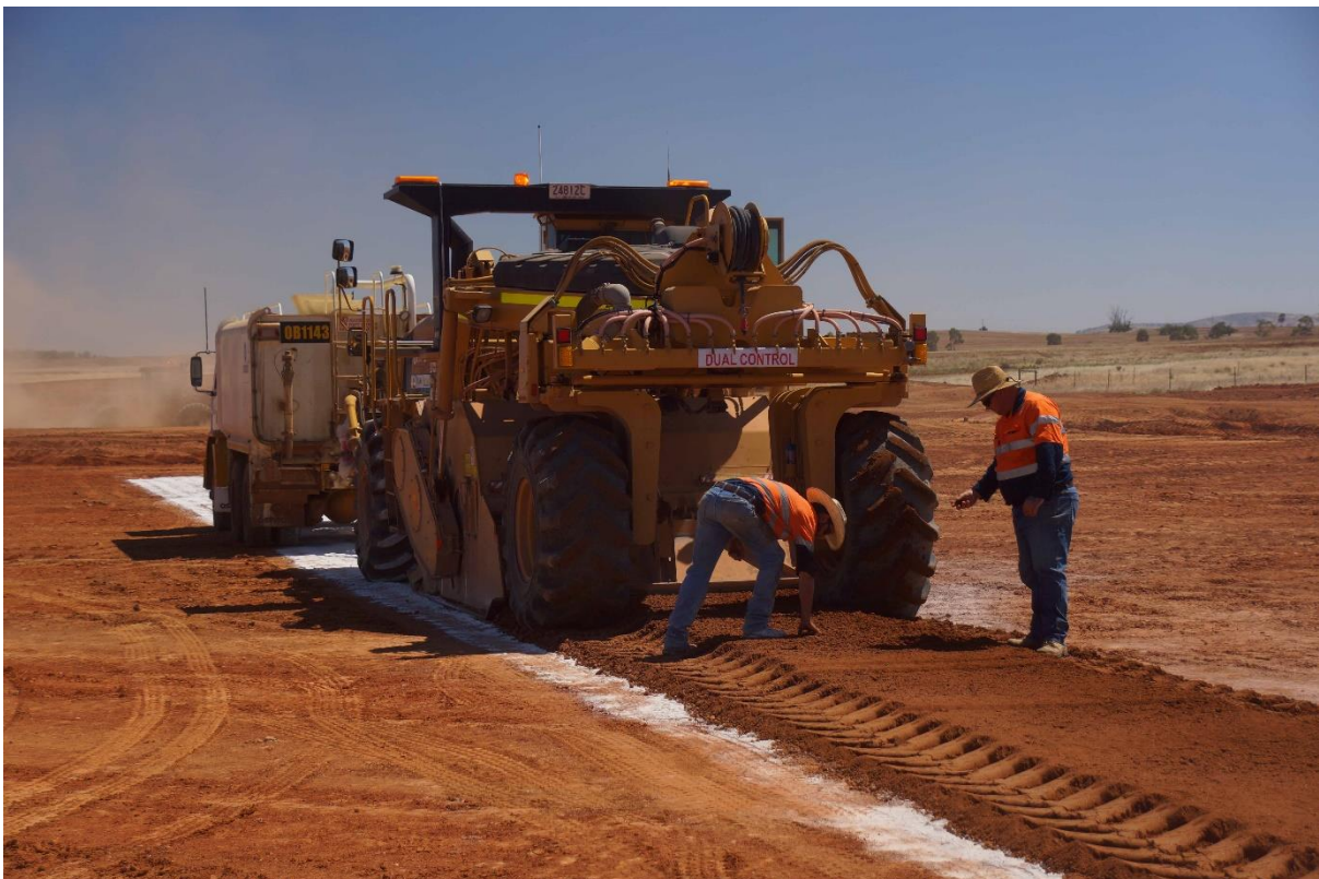
Fig. 1 Blending lime into the top 200 mm of the pen surface
