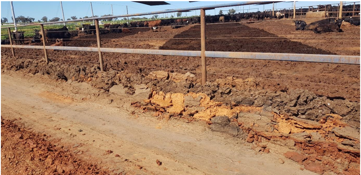
Fig. 7 Cracked surface material in alley outside stabilised Pen 90
