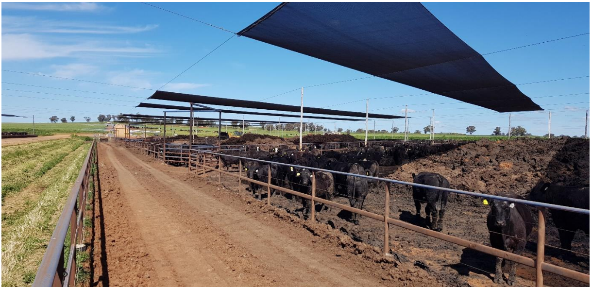
Fig. 4 Alley of control pens
