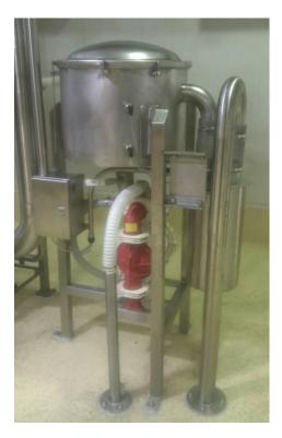
Fig.3 View of vacuum cyclone tank and diaphragm pump
