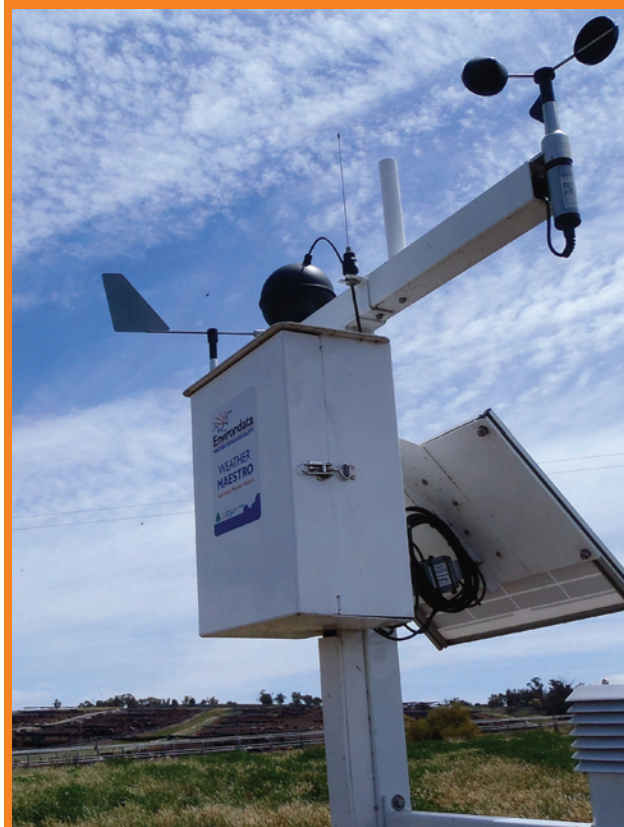
Weather Maestro with UHF link installed 2010
