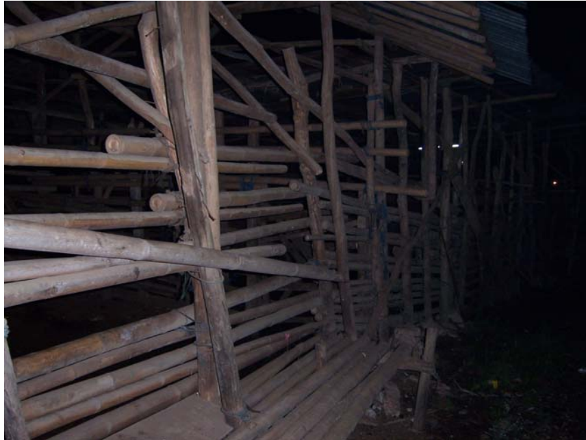
Figure 1 Section of abattoir yard in Indonesia.
