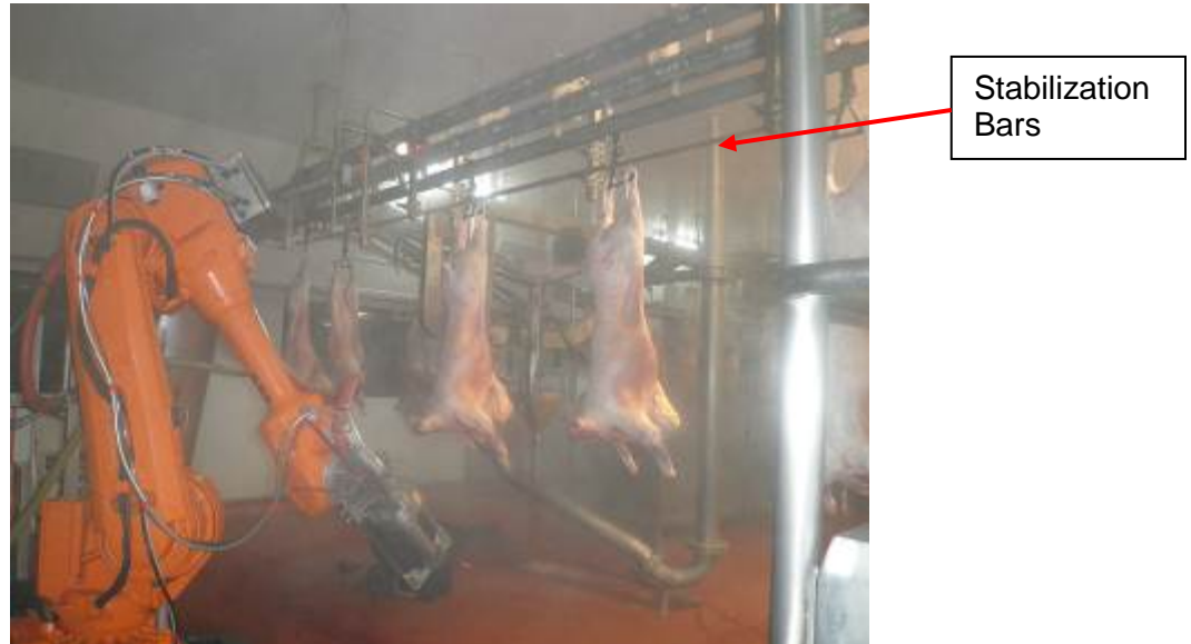
Fig.3 Stabilization bars installed at GMP.
