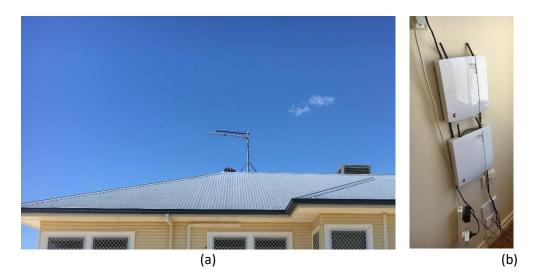
Figure 3-4. (a) An example of a dual mobile booster located on the roof of a feedlot office, and (b) the internal router boxes used to (internally) link office desktops. Note the mobile link is facilitated by a Yagi antenna. A second Yagi (directly beneath the first) is used for the point-to-point link (Wi-Fi) to an Induction shed
