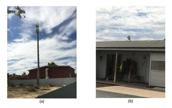
Figure 3-18. (a) NBN fixed wireless tower in a rural town and (b) fixed wireless antenna (diamond shaped) on a nearby feedlot office (4 km away).
