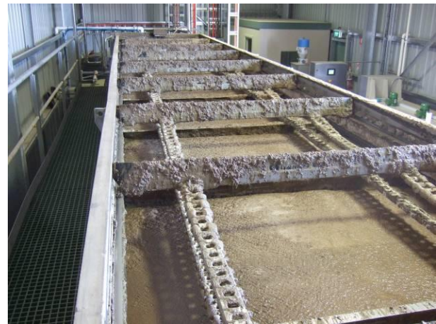
Photo 2: Float removal chain on new DAF
