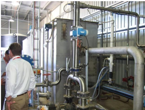
Photo 1: Elevation of new DAF
