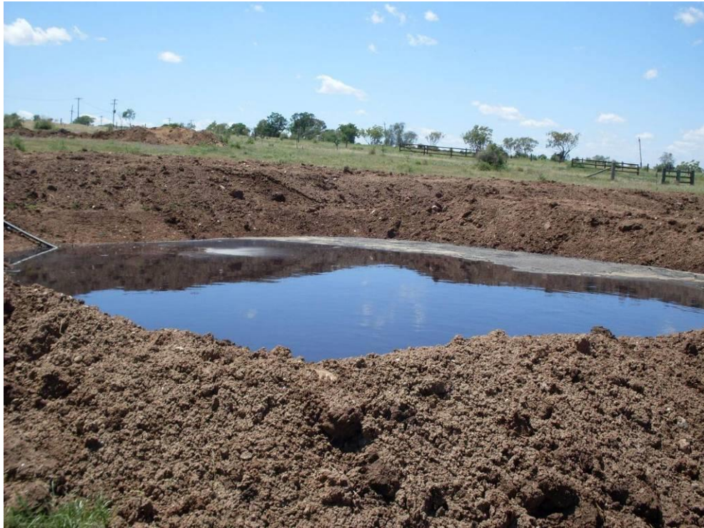
Effluent pond 1 at Jimbour Butchery
