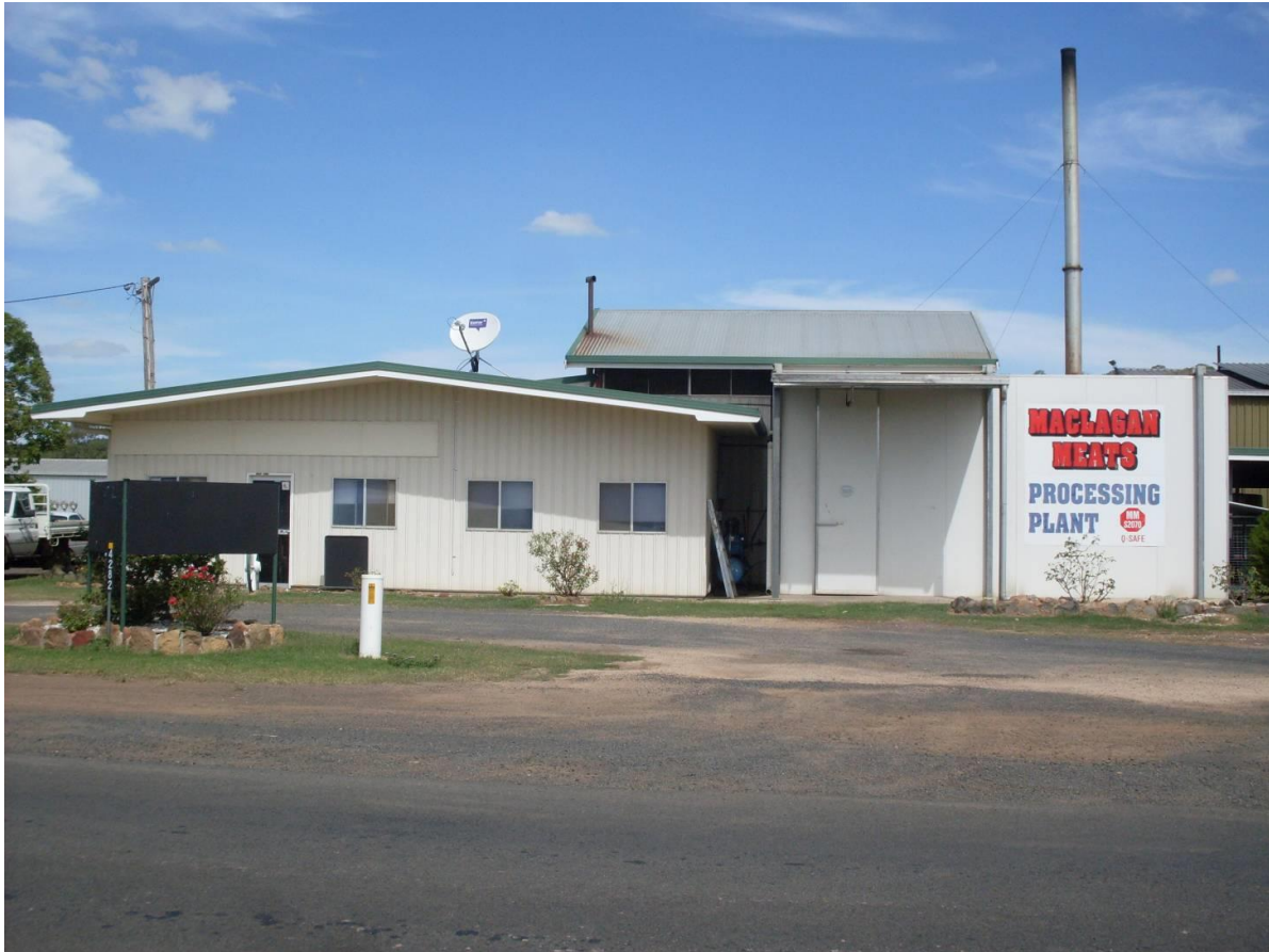
View of Maclagan Meats processing plant from road
