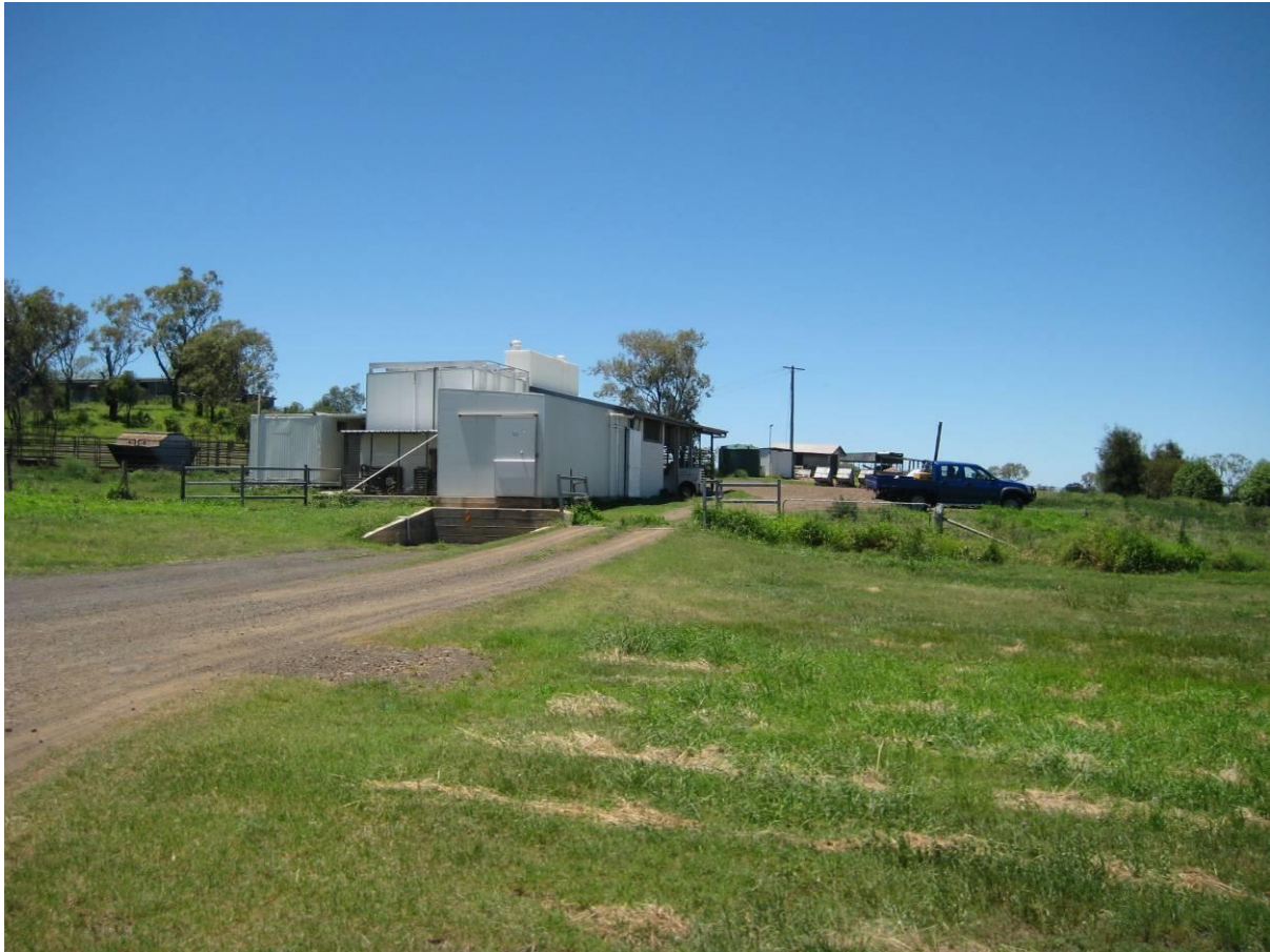
View of Jimbour Butchery from road
