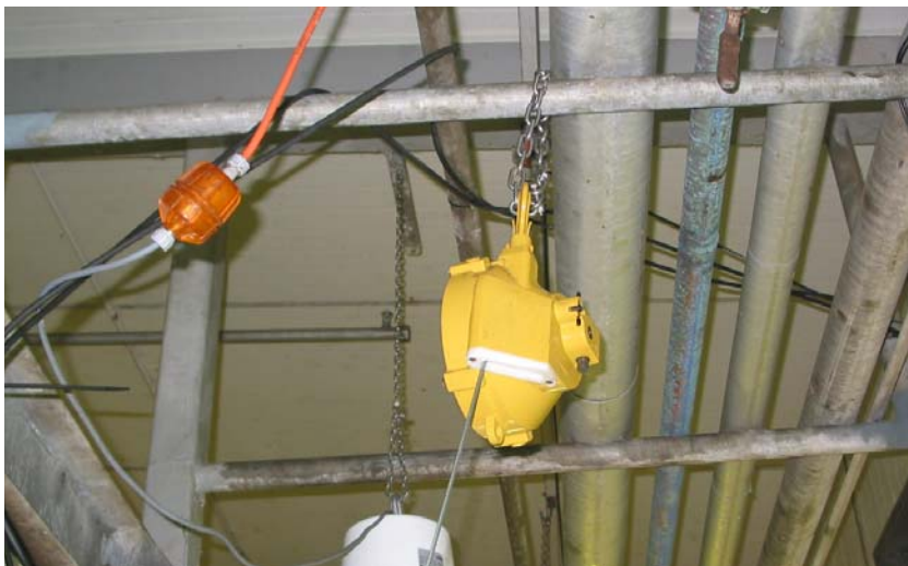
Figure 2: View of the counterbalance connection at Beef City
