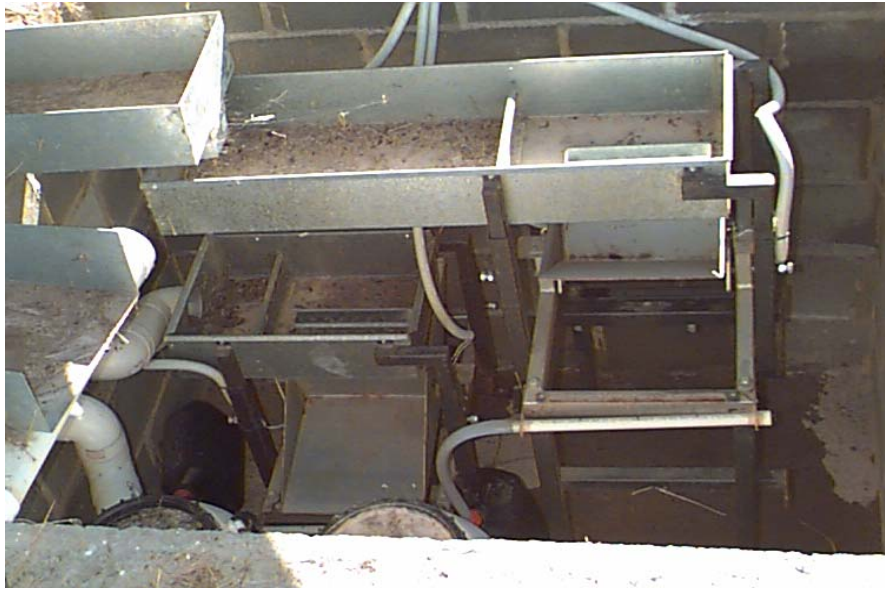
Figure 6: Tipping bucket instrumentation in pit for surface and subsurface water flows.
