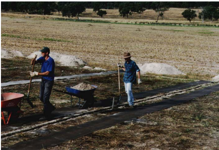
Figure 5: Installation of conveyor belting (July 1997) between plot boundaries.
