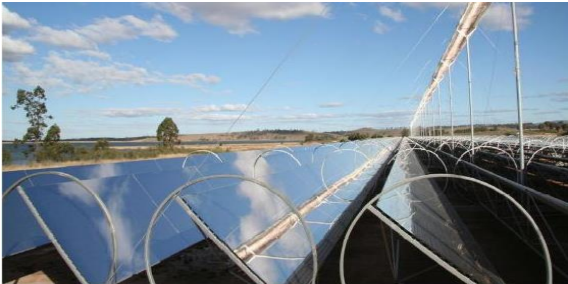
Figure 7 - Compact linear Fresnel. Source: Ausra.
