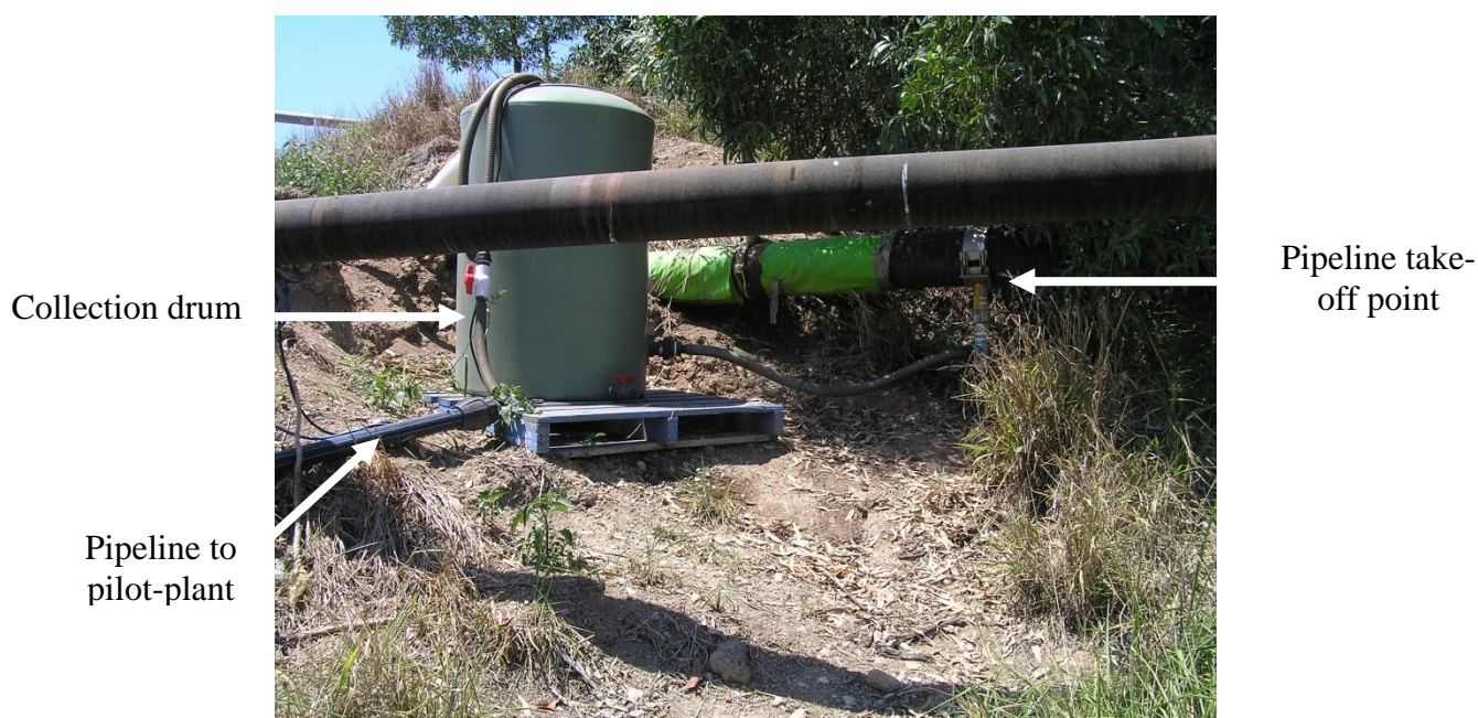
Figure 2.4: Pilot-plant take-off line and collection drum.
