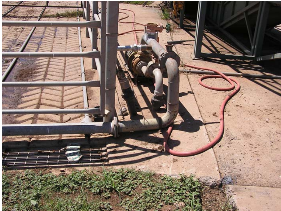
Photo 4 Flooring, pipework and drain of a feedlot cattle wash
