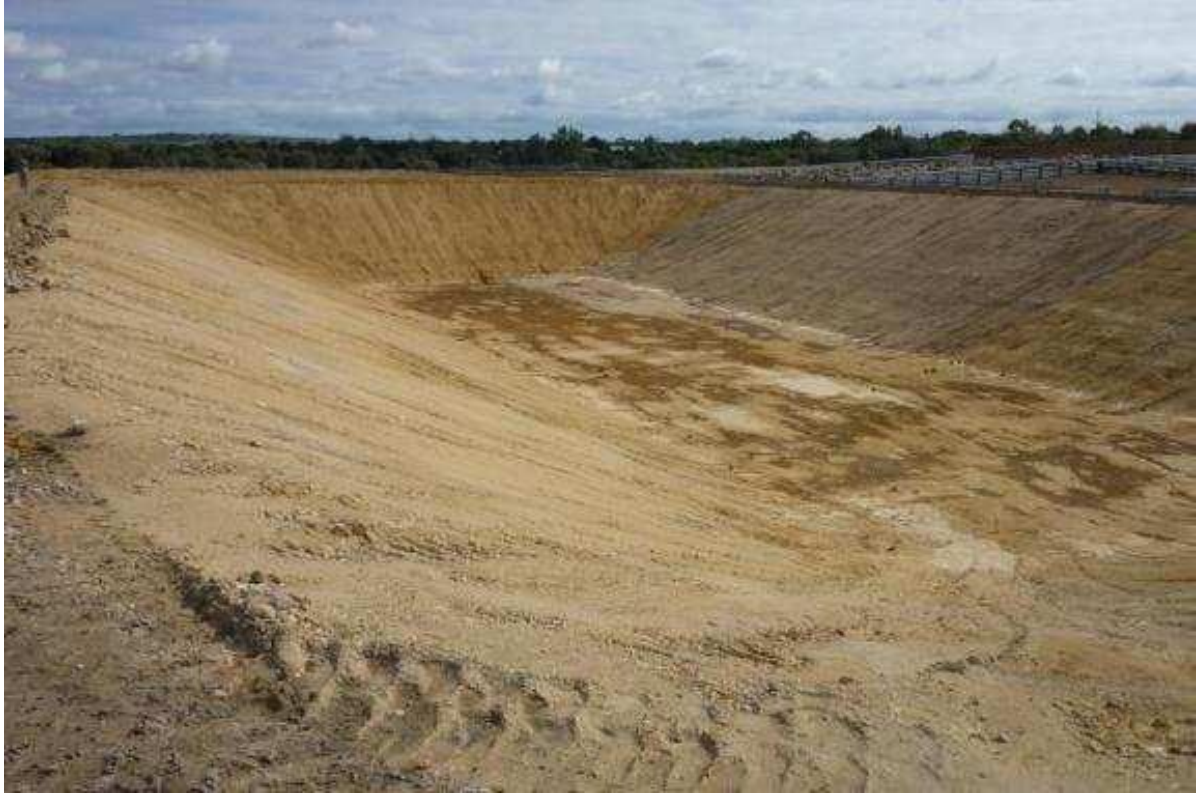
Figure 16: Bulk excavation of eastern CAL
