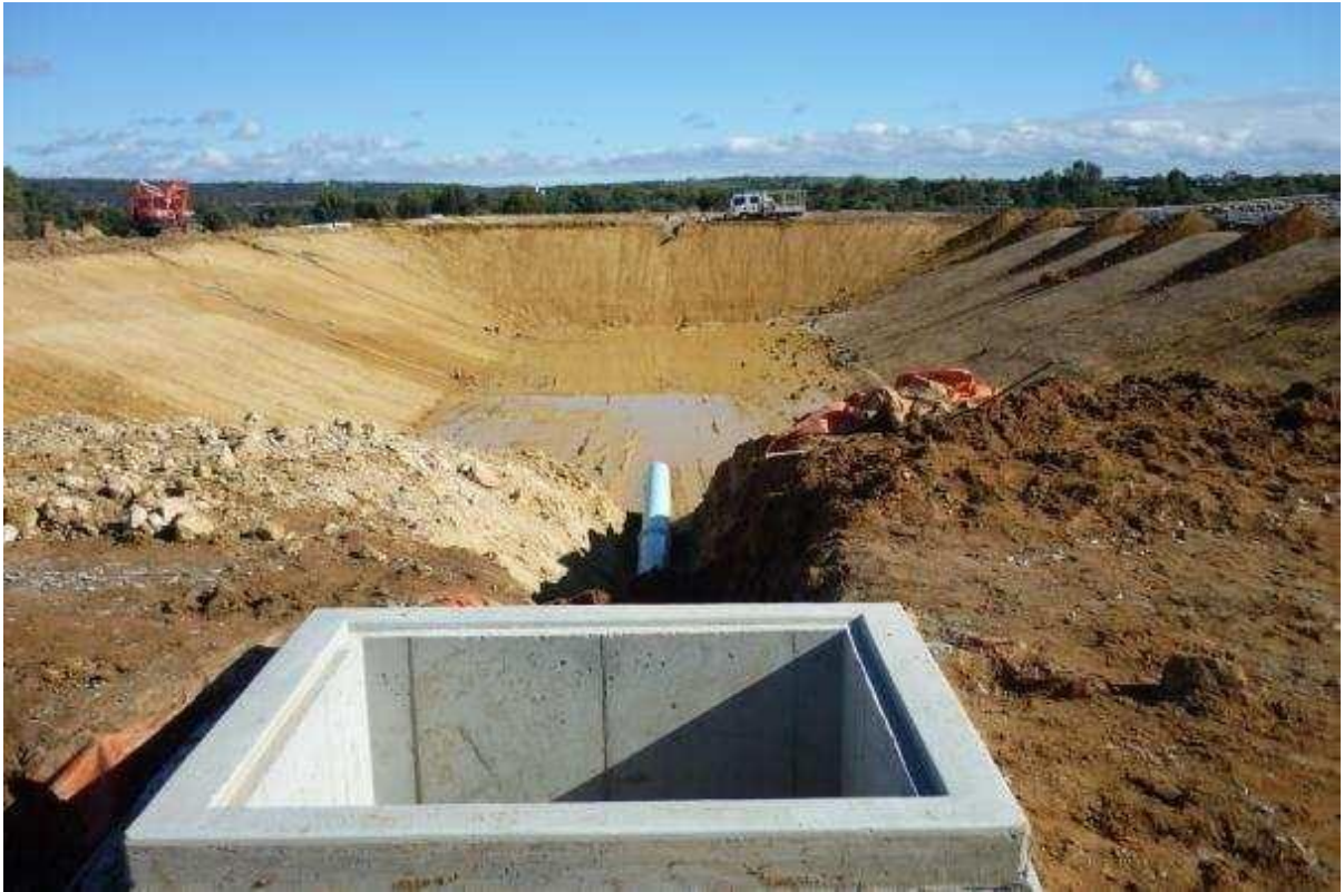
Figure 26: Eastern CAL outflow weir
