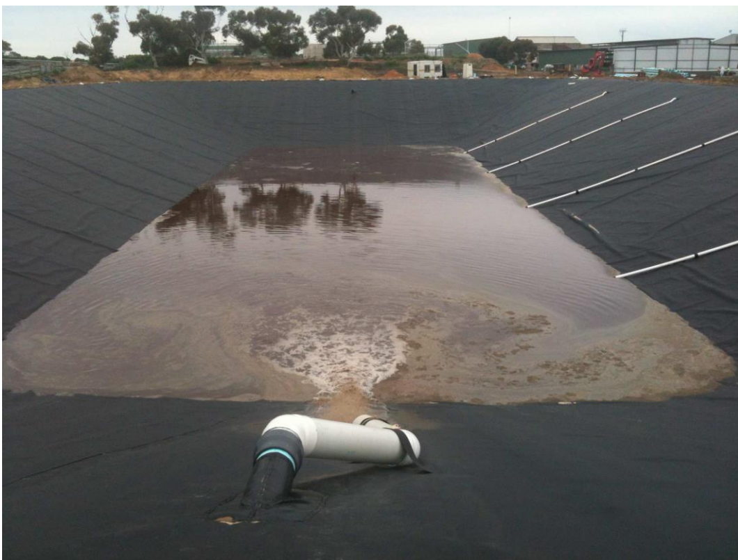
Figure 29: Inlet to eastern CAL during initial filling
