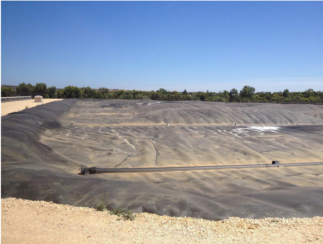
Figure 31: Western CAL showing some biogas generation
