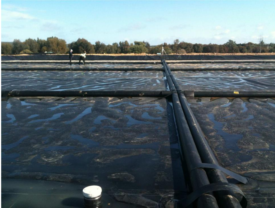
Figure 20: Cover weigh down system during construction
