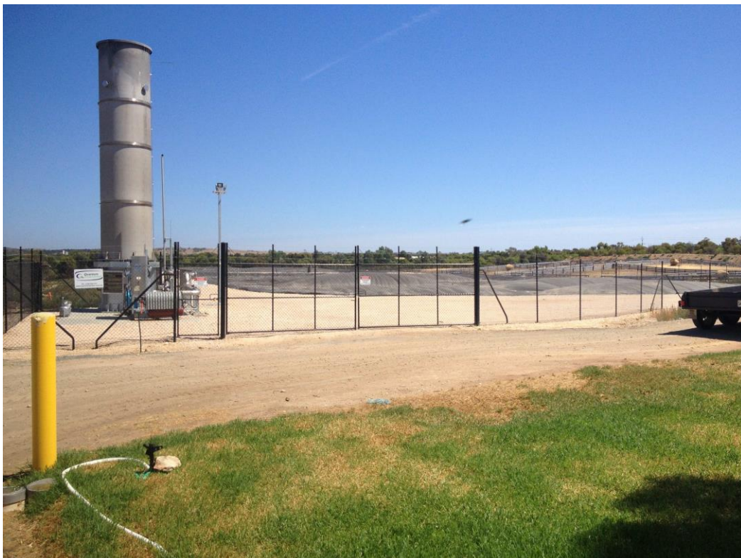
Figure 34: Flare and security fence
