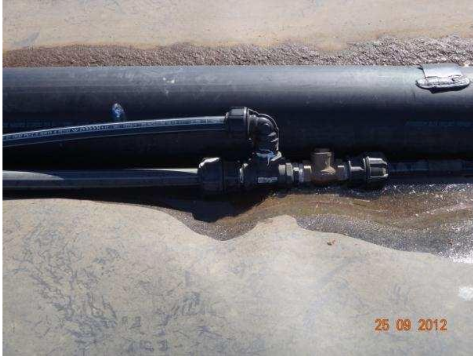
Figure 19: Rainwater removal system
