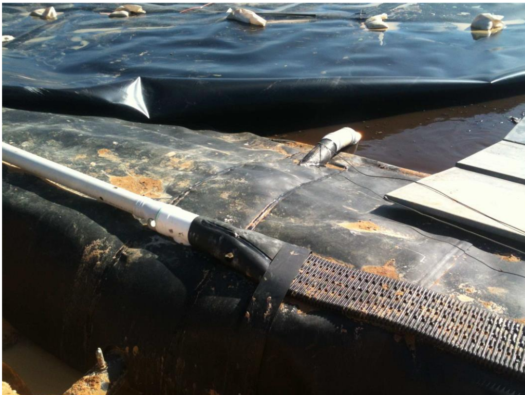
Figure 10: MegaFlo gas collection pipe
