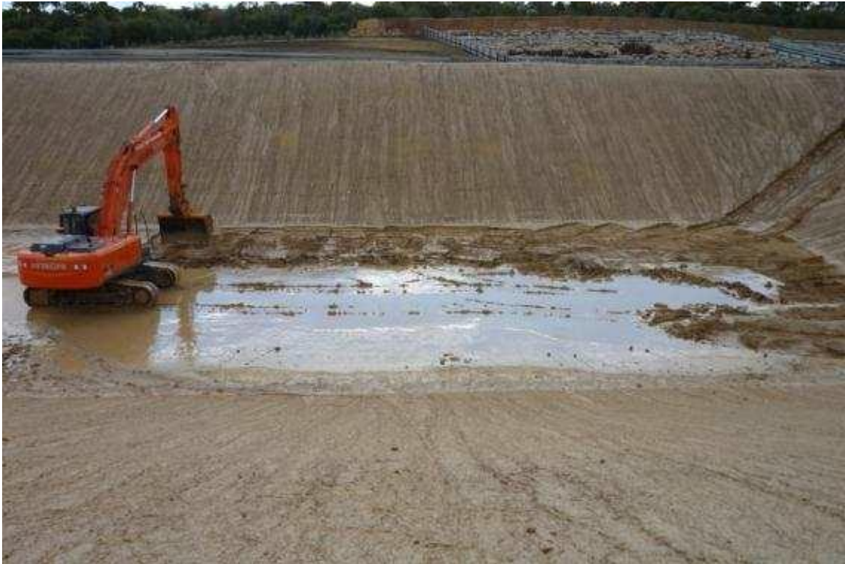
Figure 17: Re-working earthworks following rainfall
