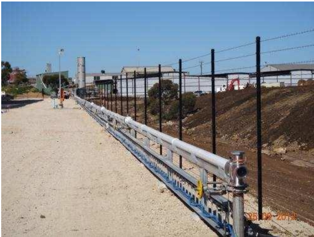
Figure 30: Pipe bridge located on outside of embankment
