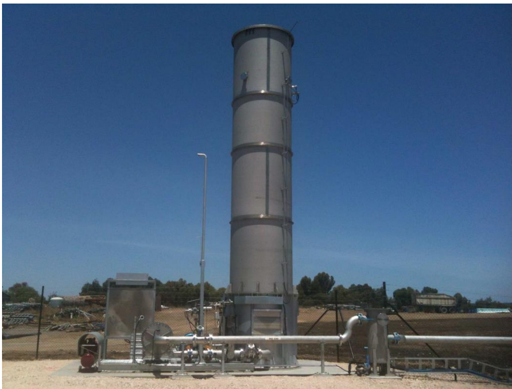
Figure 15: Installed gas train and high temperature flare
