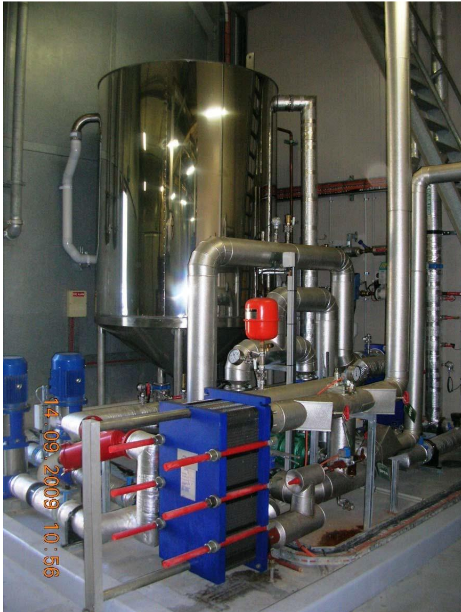
Photo A1.1 – Water tank – water-Glycol HEX and Glycol-NH3 HEX
