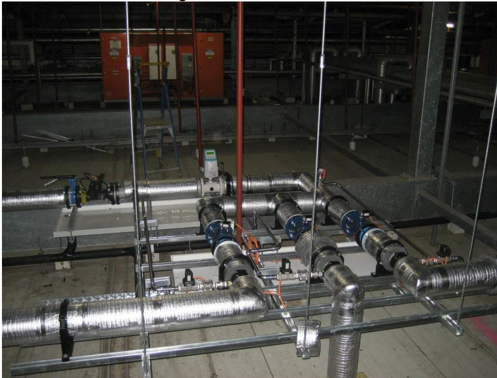
Photo A1.4 Above Ceiling Valve station
