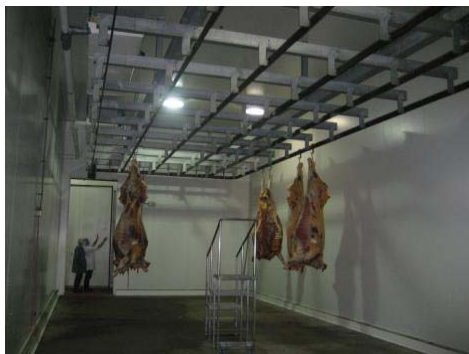
Image of ECT Chiller prior to install
