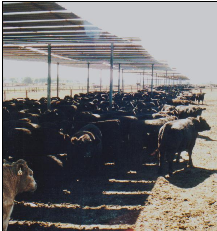
Plate 1. Galvanised Shade Structure at Feedlot A.
