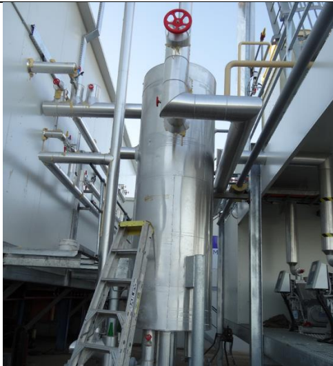
Figure 13 - Inter-Cooler
