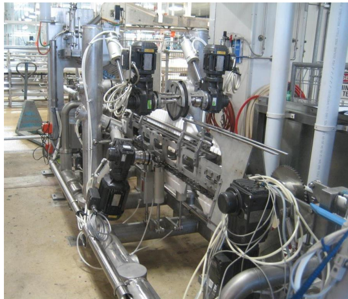
Figure 3: Chine boning station being installed.
