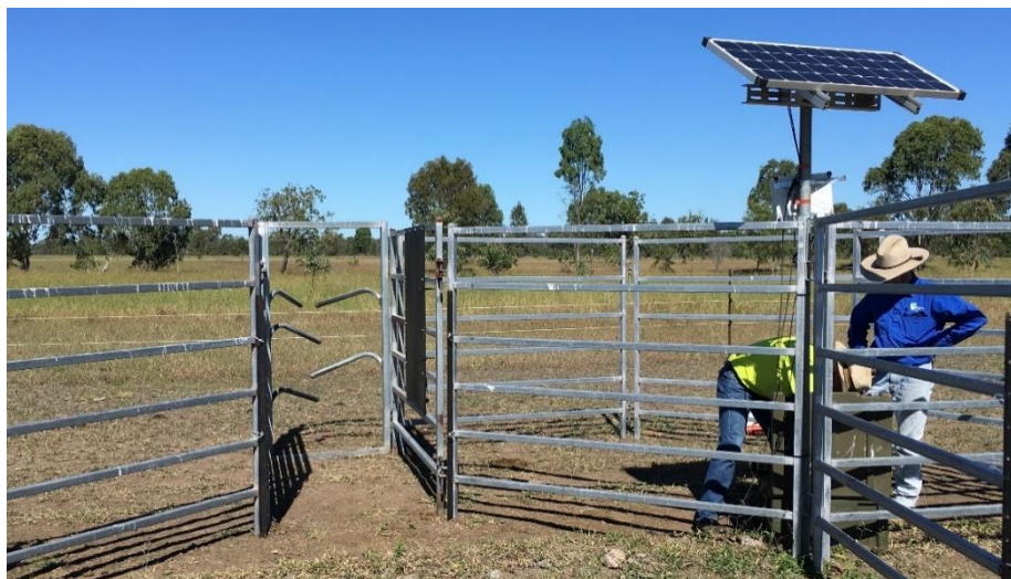
Fig. 14. RFID reader and solar panel being installed at the exit of the left draft pen
