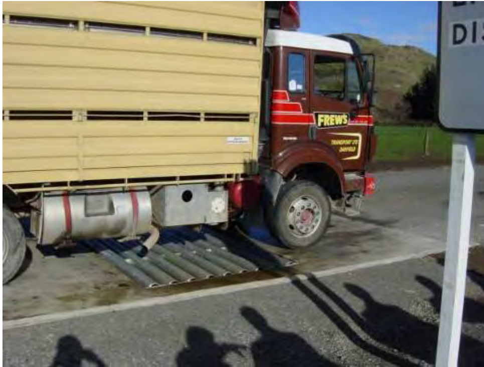
Photograph 6 – Stock truck dumping effluent over grate (New Zealand)
