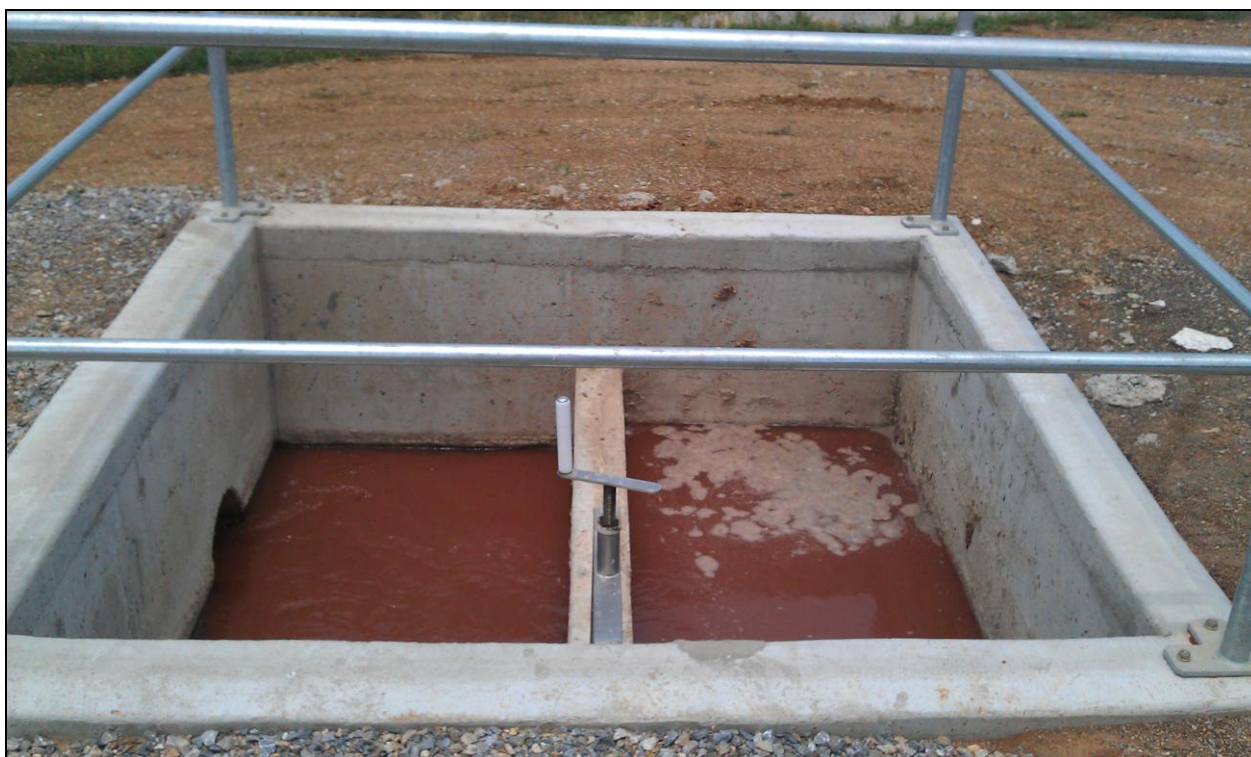
Photo 3.4 – Abattoir A CAL system: Outlet wastewater collection point
