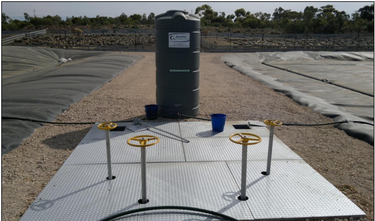
Photo 3.9 – Abattoir C: Inlet wastewater collection point
