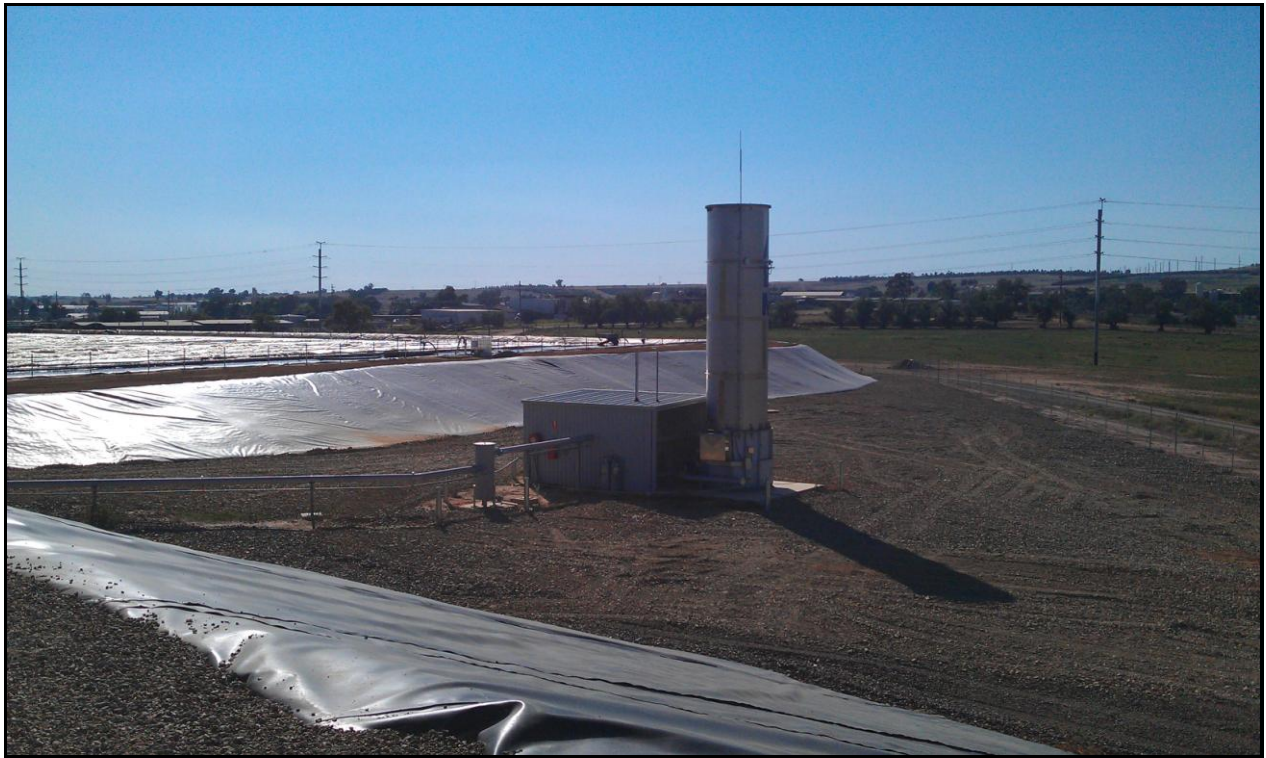
Photo 3.11 – Typical biogas flare system
