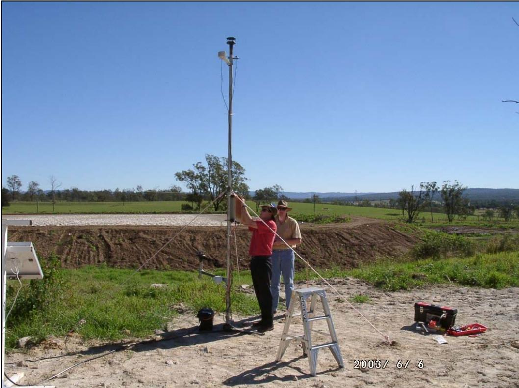
**Figure 7: Weather station being installed on site (looking north west)**
