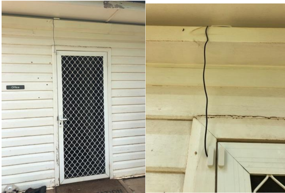
Figure 12: Office door sensor
