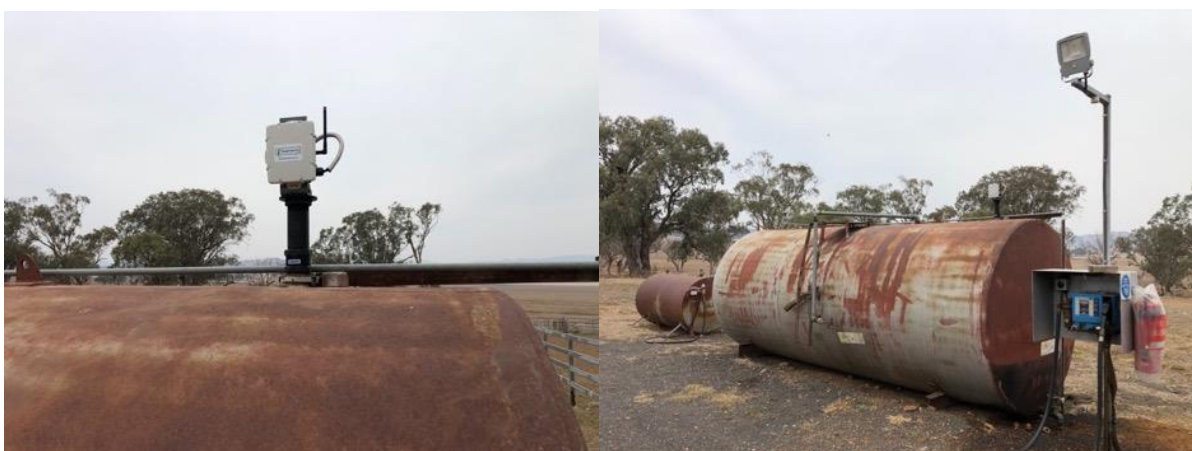
Figure 9: Diesel fuel tank sensor
