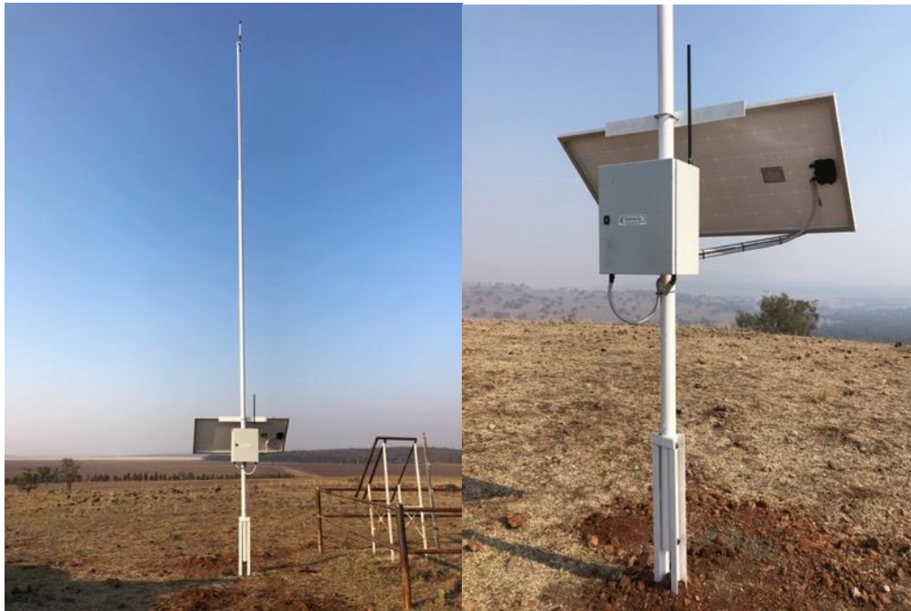
Figure 3: Windy station gateway installation photos
