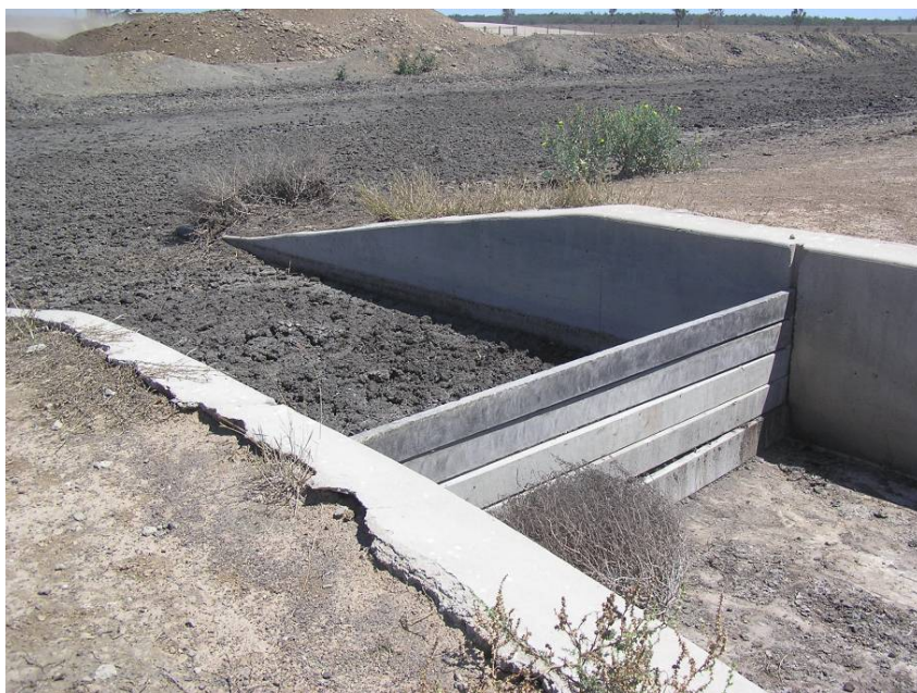
PHOTOGRAPH 7 - TYPICAL SEDIMENTATION BASIN AT A FEEDLOT
