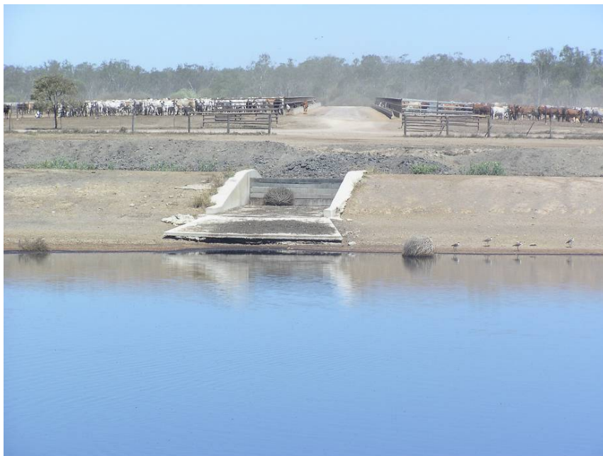
PHOTOGRAPH 6 - TYPICAL FEEDLOT RUNOFF HOLDING POND
