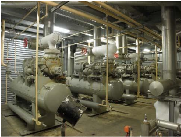
Figure 5: New Plant Screw Compressors. Figure 6: New Plant Evaporative Condensers.
