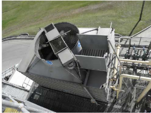
Figure 5: New Plant Screw Compressors. Figure 6: New Plant Evaporative Condensers.
