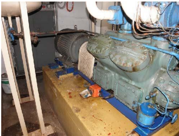
Figure 1: R22 Reciprocating Compressor.
