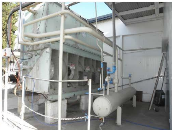
Figure 2: R22 Evaporative Condenser.
