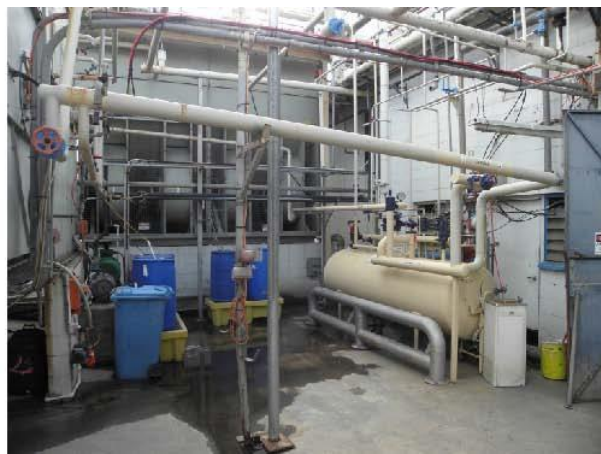
Figure 4: Old Plant Evaporative Condensers.
