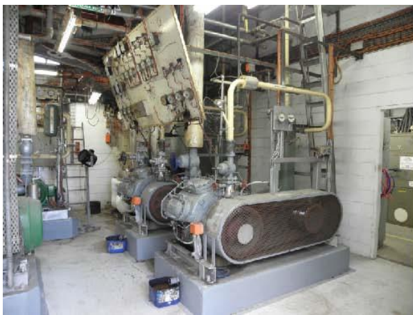
Figure 3: Old Plant Reciprocating Compressors
