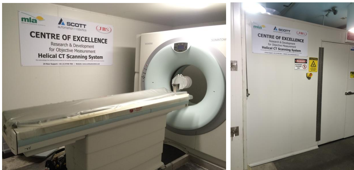
Figure 5 - Completed CT room inside (left) and outside (right)
