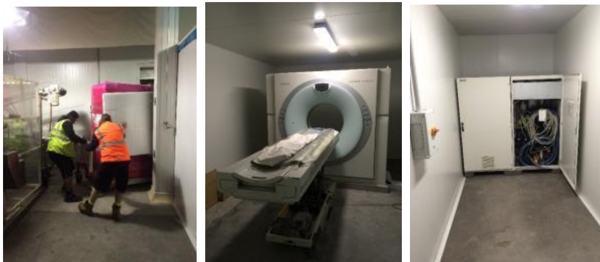
Figure 4 - Installation of CT scanner (left, middle) and electrical rack in control room (right)
