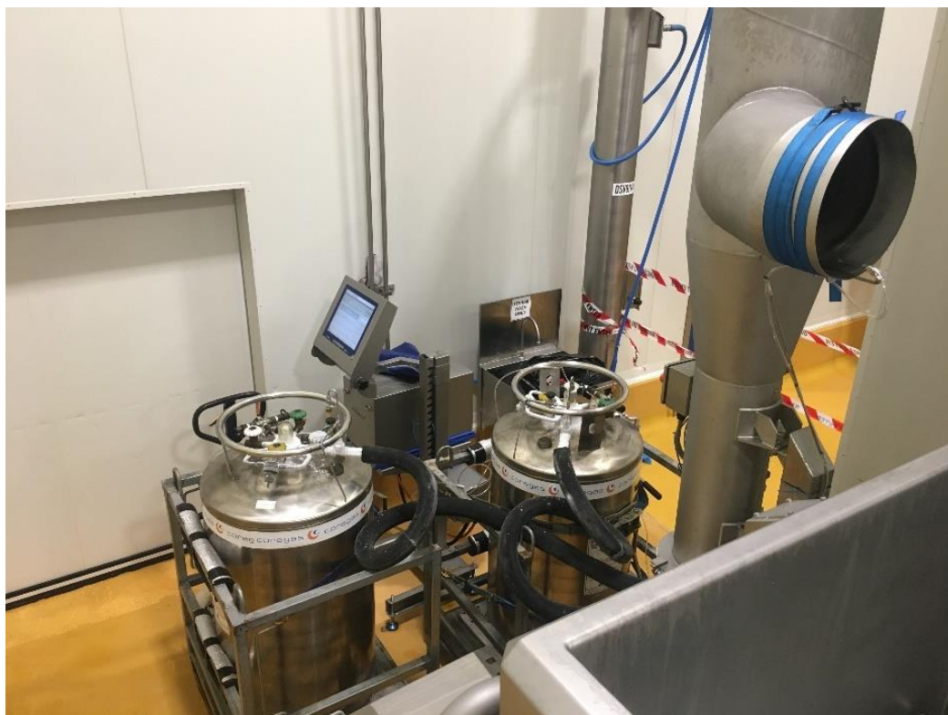
Photo 2: Vacuum jacketed liquid nitrogen vessels.
