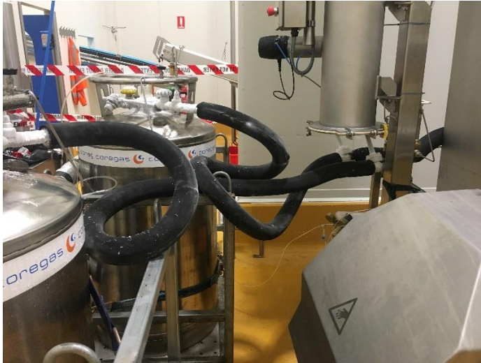
Photo 3: Nitrogen vessels and supply piping.
