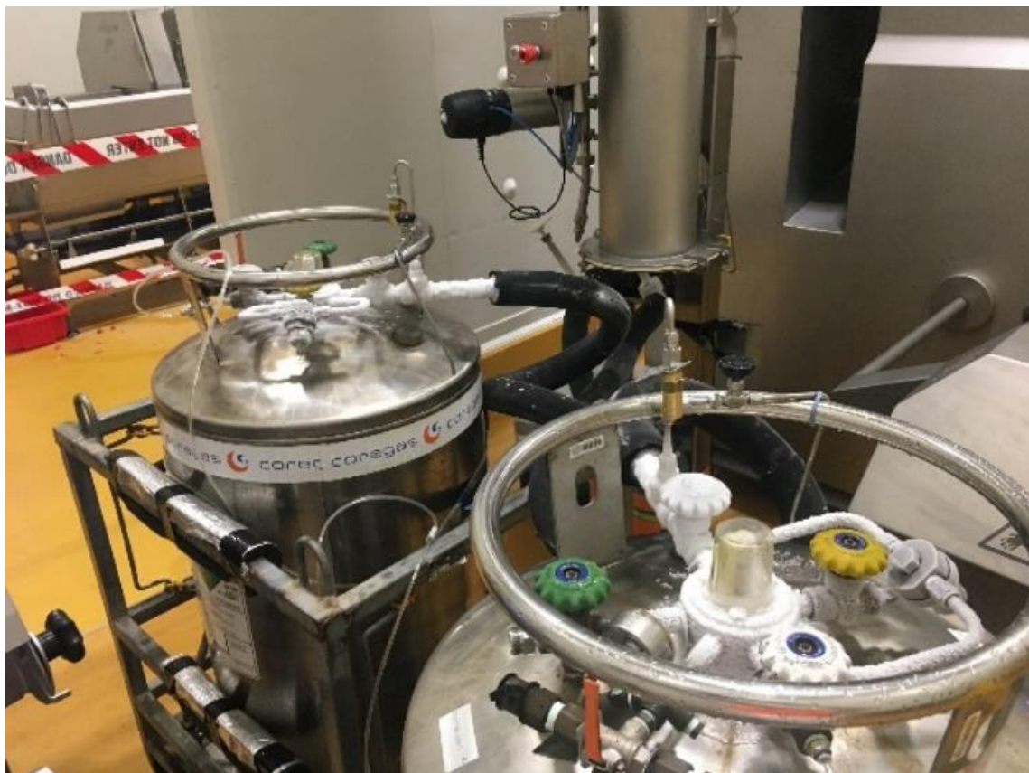
Photo 4: Safety perimeter around nitrogen vessels and mixer.
