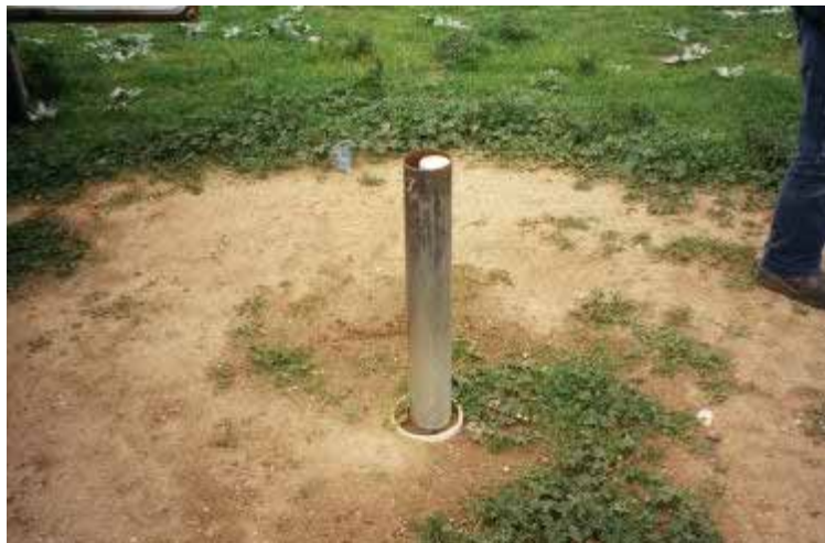
Groundwater bore protected against cattle damage
