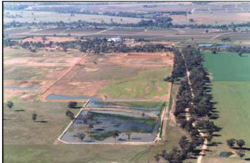
Aerial view of a processing plant and wastewater treatment
