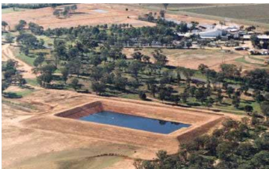
50 ML wet weather storage dam
