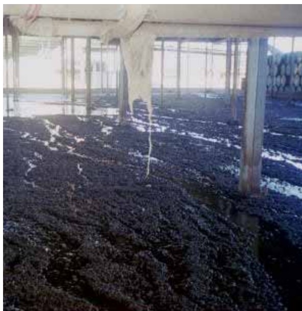
Manure under the floor of a sheep shed
