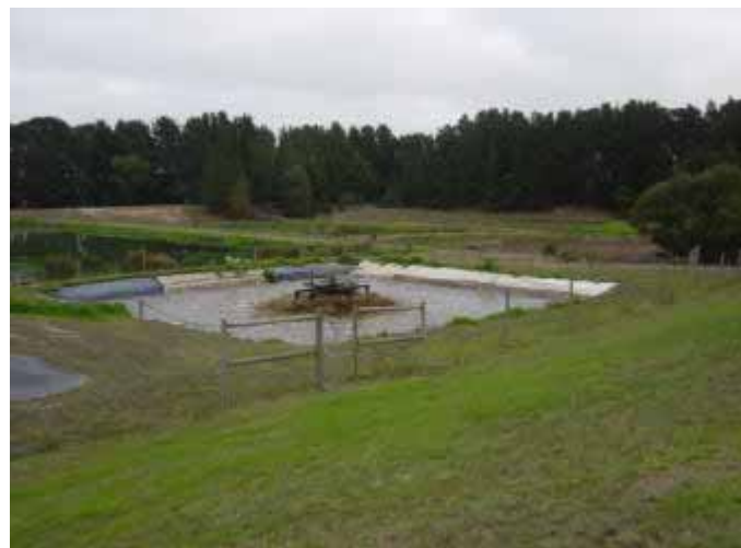
Sequencing Batch Reactor
