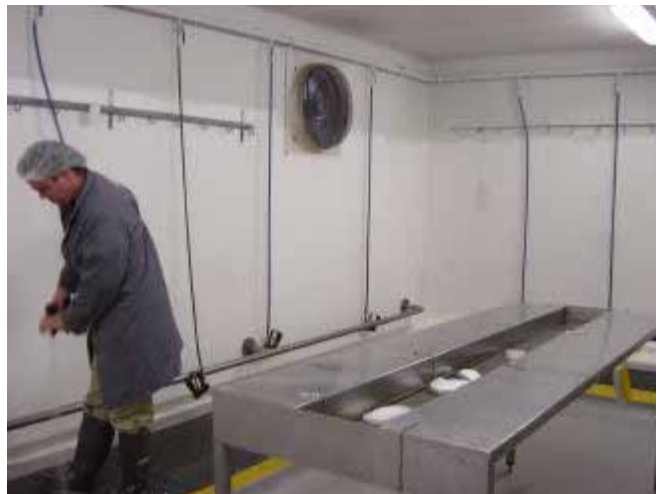
Boot washing facility
