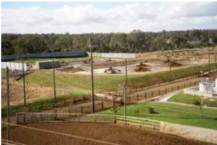
Aerial aspect of a Wastewater Treatment Plant
