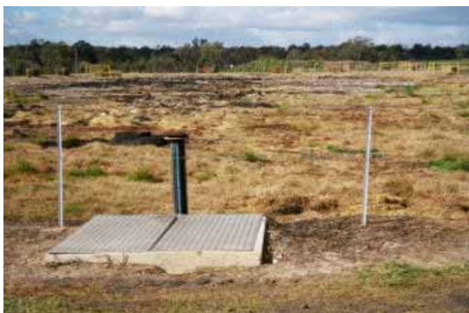
Anaerobic pond with a naturally formed crust
