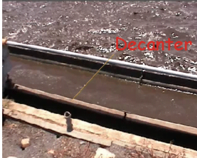
Figure 4. SBR 4A decanting weir of tilting plate type
