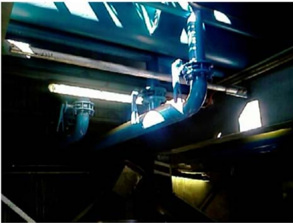
Photograph 7 - Air feed to the cake bins
