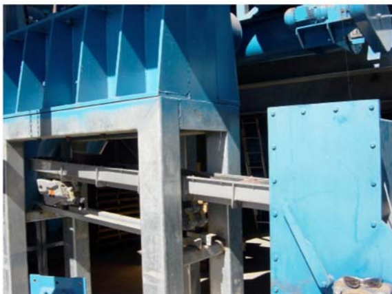
Photograph 9 - The vibrating mill discharge conveyor during construction
