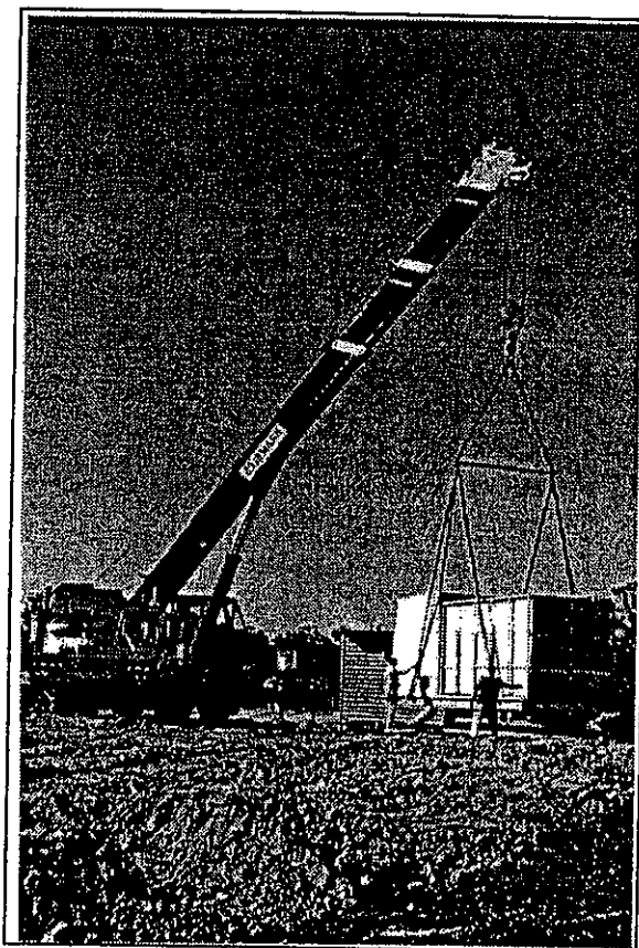
Figure 9-2: Installation of portable SBR unit at Dinmore abattoir
